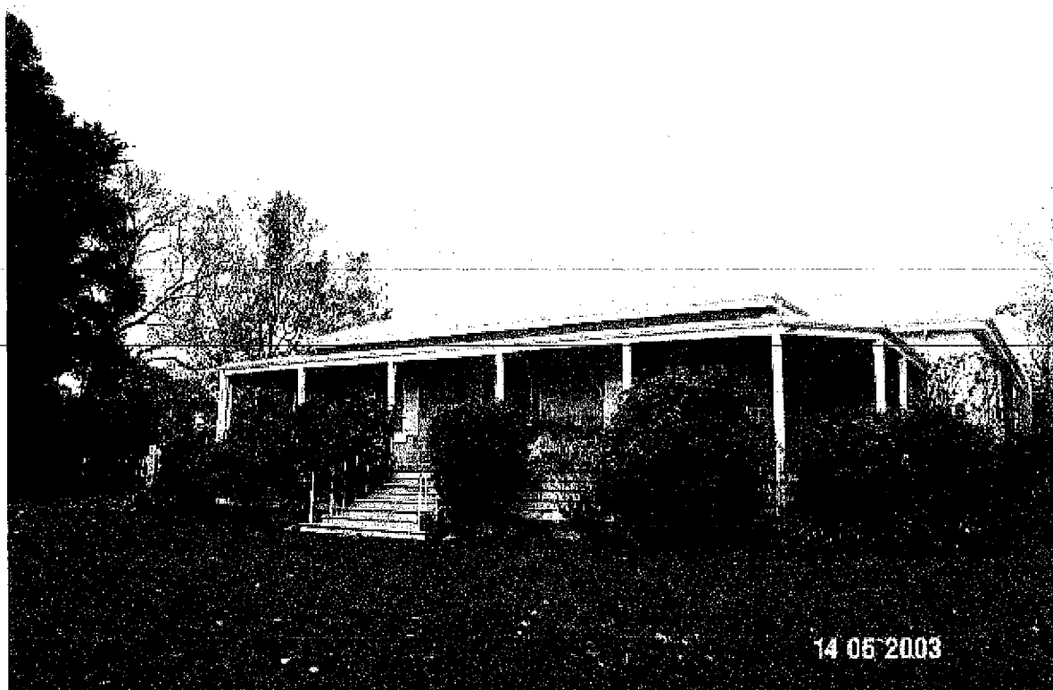
Toolang Homestead, Parkwood Road, Coleraine. Façade.
