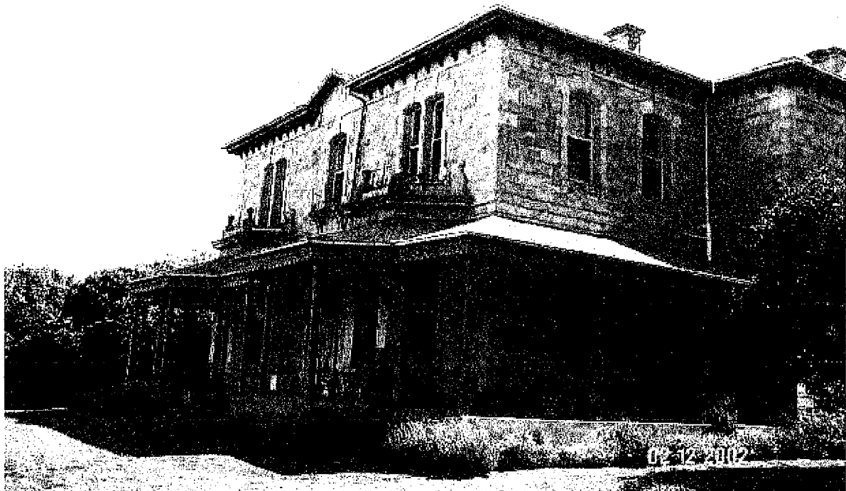
Gringegalgon Homestead, façade
