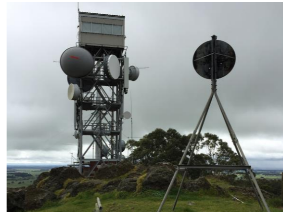
Telecommunications equipment on summit
