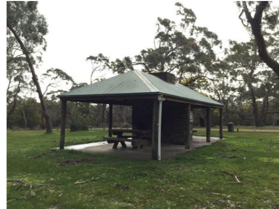
Upper Carpark, picnic shelter
