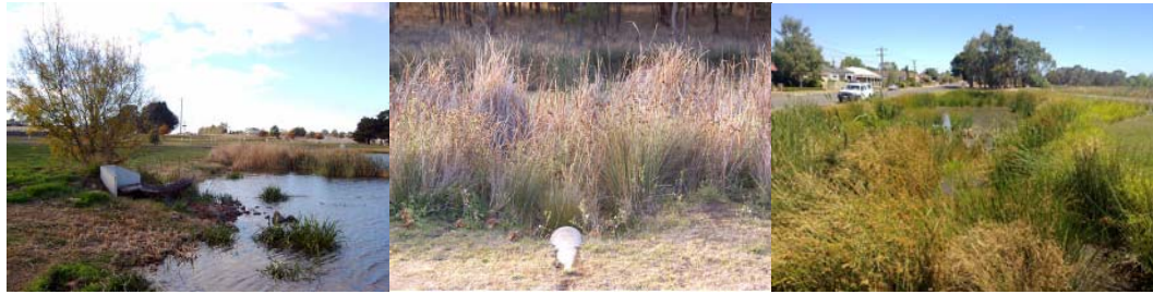
Plate 3. Examples of stormwater drains to Lake Hamilton – piped inlet (left), grass swale (centre) and the Frog Settling Pond. The pipe and grass swale photos were sourced from The Regional Development Company (2006)
