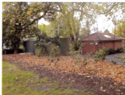
Figure 11: Toilets and water tanks
