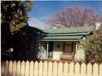
Figure 22: Former Caretakers Cottage
