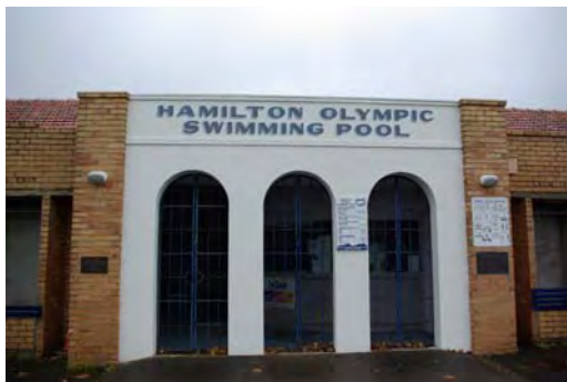
49) Main entry signage – clear from street.
