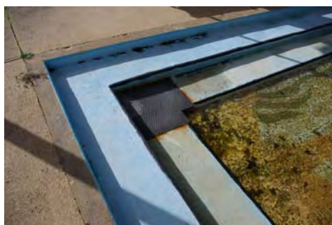
26) Grate plates – corroded. May create trip hazard. 27) Corroded plates to overflow grate to toddler's pool.
