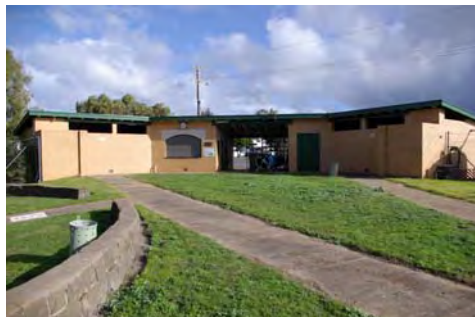
41) Signage to change rooms in poor condition.
