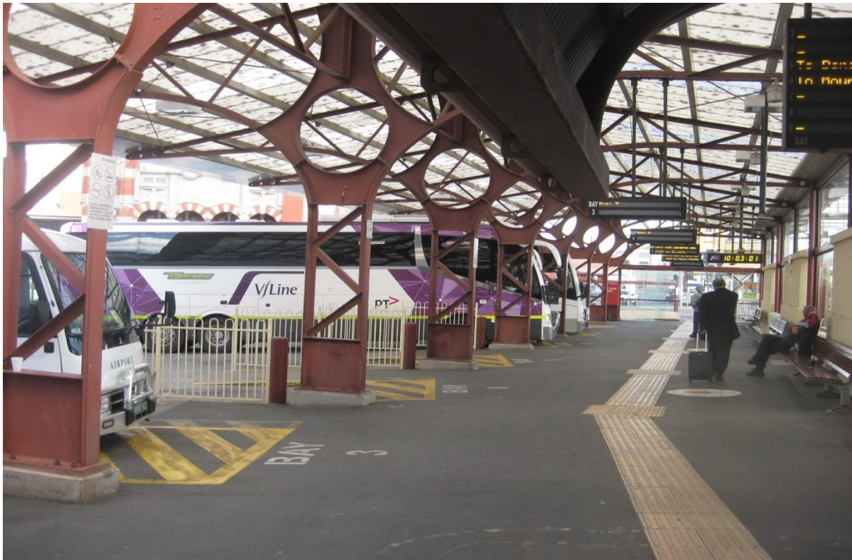
Figure 4: Road coach terminal at Ballarat Station
