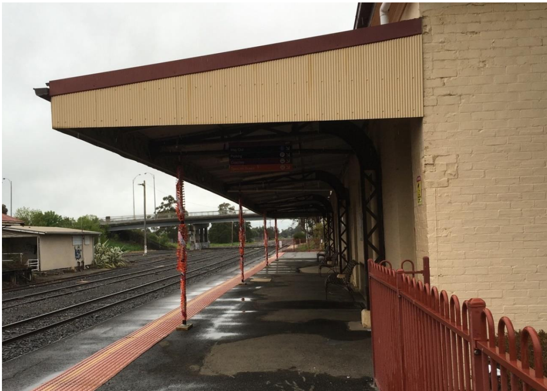
Figure 22: Horsham Station platform and building
