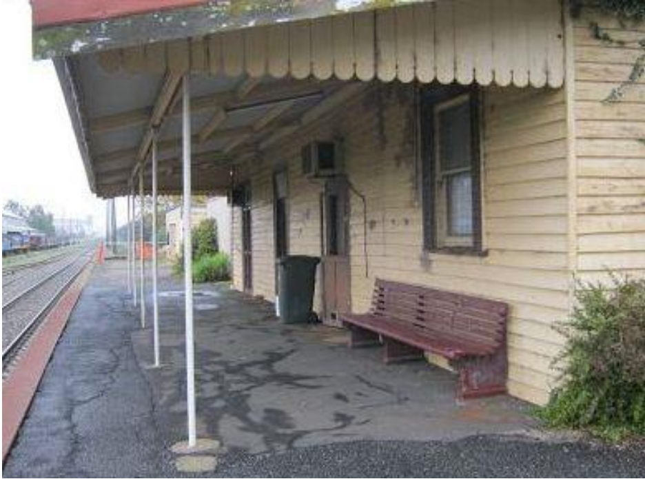
Figure 21: Murtoa platform and station building showing present somewhat dilapidated condition
