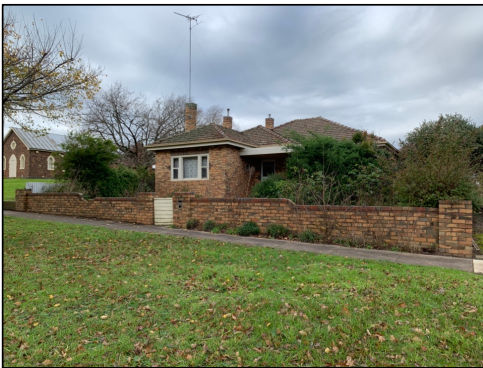
Figure 13 Existing dwelling at 122 Lonsdale Street to be demolished.
