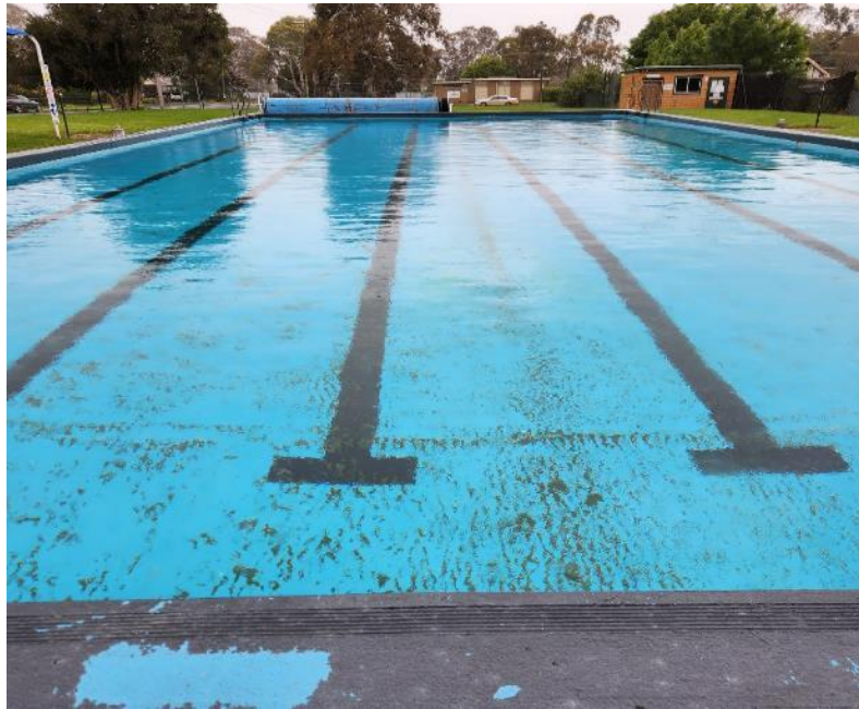
Image 7 : Main pool, Looking north to deep end.
