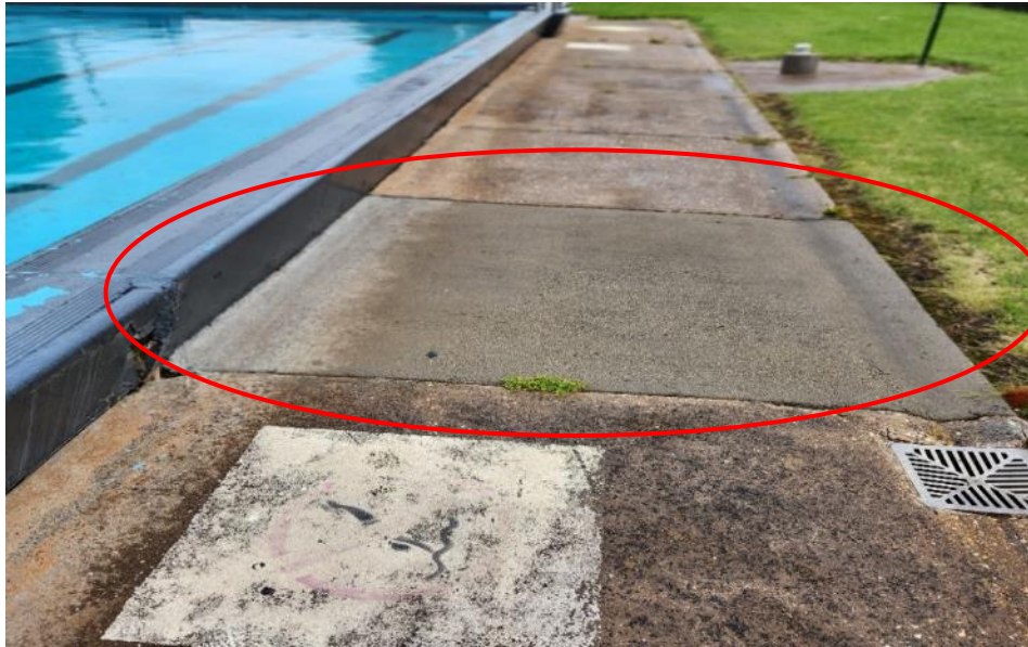
Image 14: Main pool. 'Bulging' expansion joint in previous image probably linked to this concourse panel replacement.
