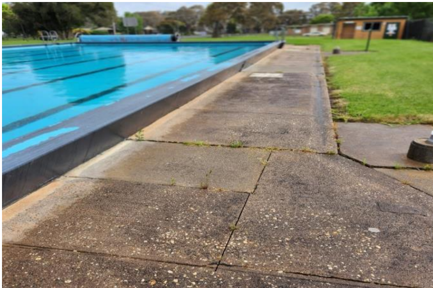
Image 22: Concourse, east side, looking N
