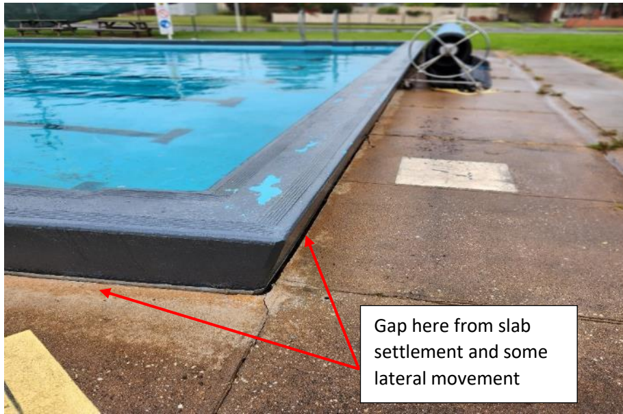
Image 23: Concourse at deep end of pool. Note gap here between hob and slabs
