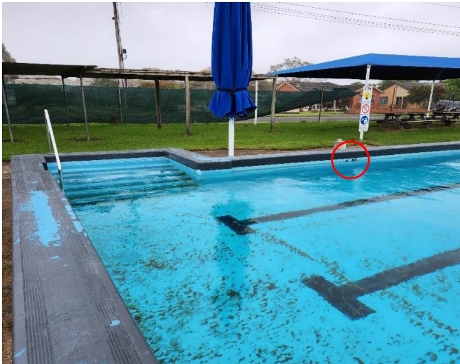
Image 8: Main pool, Shallow end steps. Looking west. Depth signs partially obscured.
