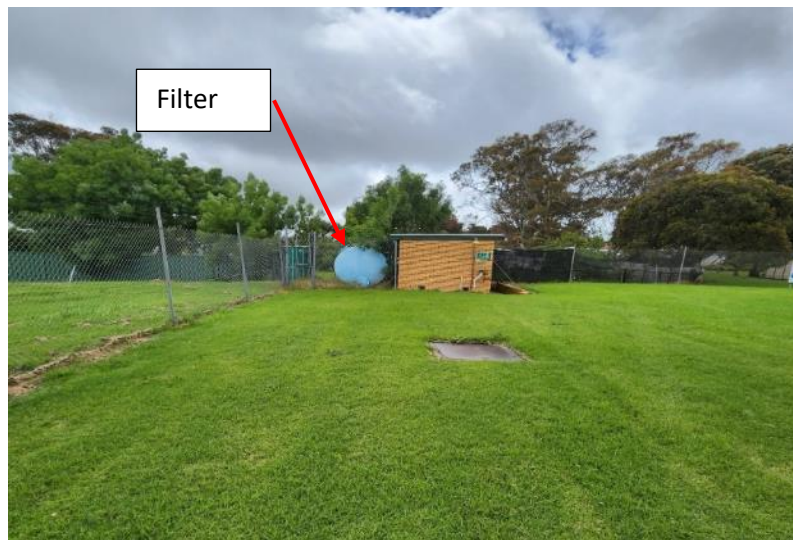
Image 25: Water Treatment Plant shed and pressure filter outside. Looking east
