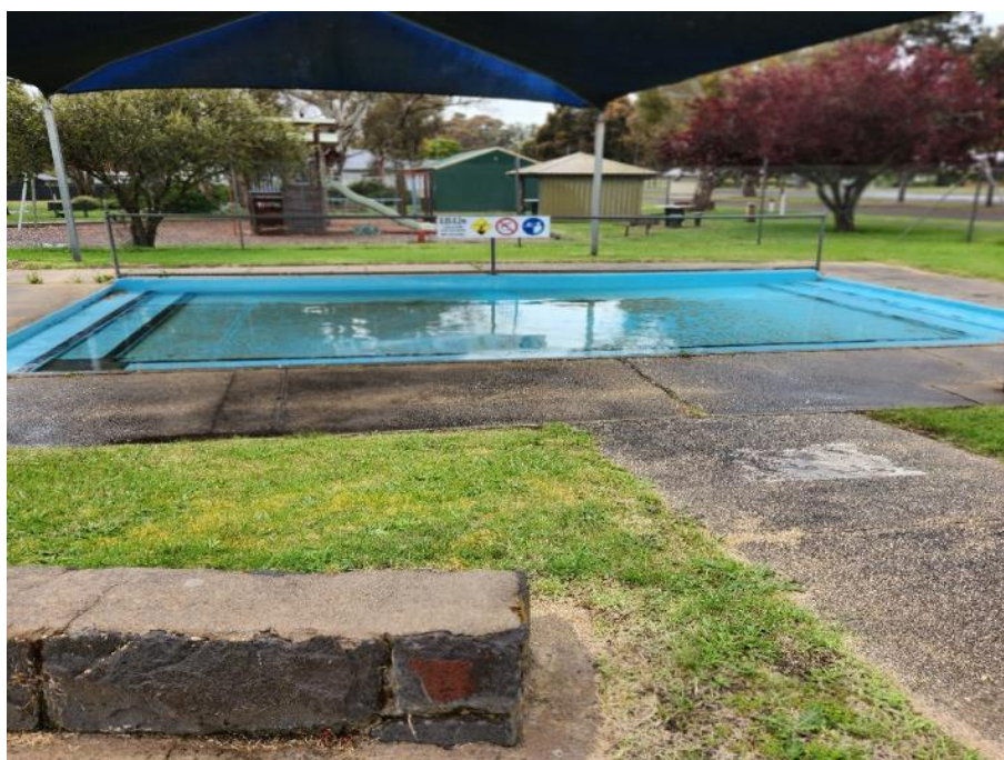
Image 17: Toddler's Pool. Looking east
