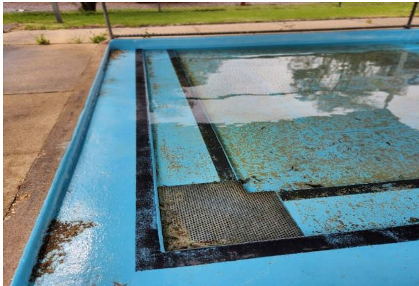
Image 18: Toddler's Pool. Soiled Water outlet grate, NW corner
