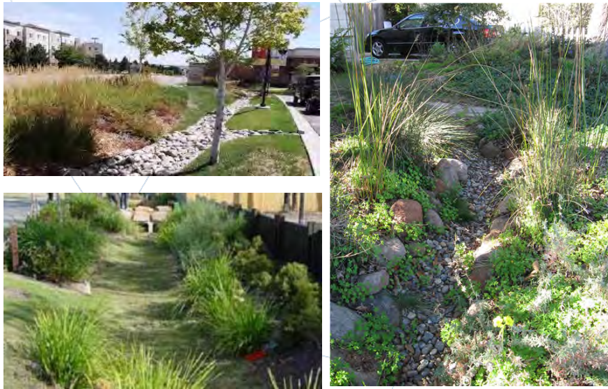
FIGURE 22: EXAMPLES OF GRASSED SWALE DESIGNS
