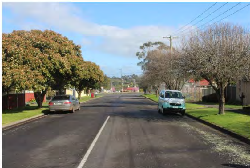
Photograph 6: Collins Street, view to the south west towards Pope Street
