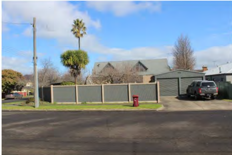
Photograph 11: 17 -19 Stephen Street, Stephen Street frontage
