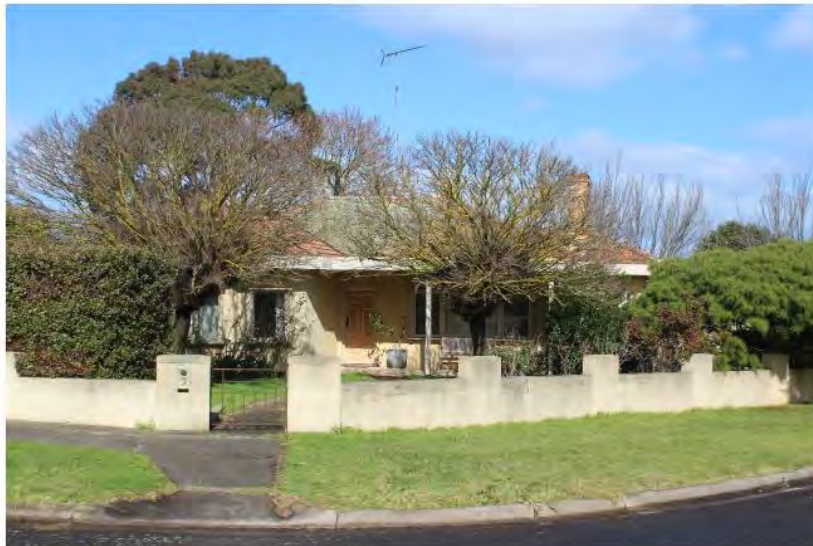
Photograph 16: 7 Dryden Street (Cnr. Collins Street), diagonally opposite the application site
