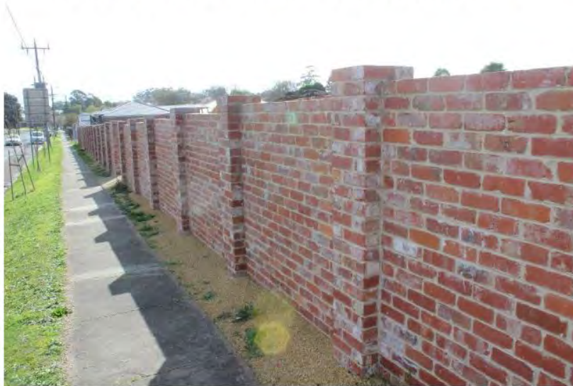
Photograph 4: Pope Street frontage immediately north of the application site
