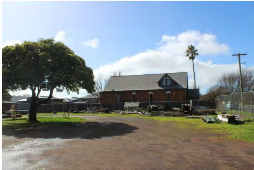
Photograph 5: Adjoining dwelling to the east of the application site (i.e., 17-19 Stephen Street)
