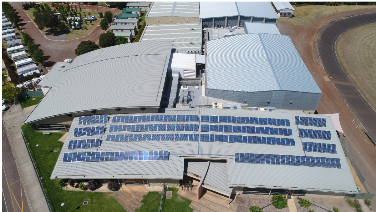
Figure 5. 60 kW solar PV generation at HILAC
