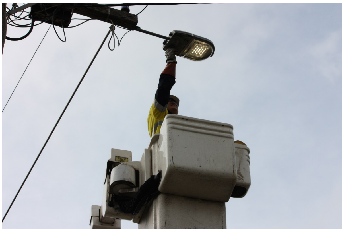
Figure 11. Replacement of mercury vapour street lights with LED
