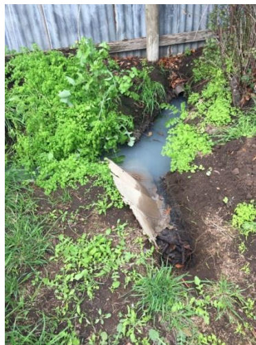
Figure 6: Effluent disposal at surface level
